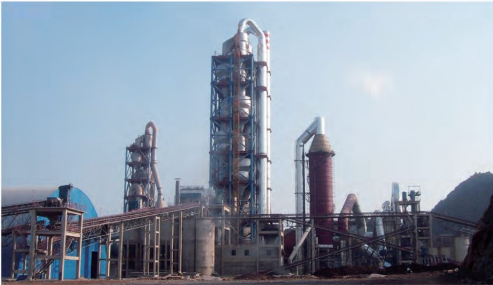
越南缘河水泥公司1500t/d+5000t/d熟料生产线 1500t/d+5000 t/d Clinker Production Lines at Duyen Ha Cement Company Vietnam
