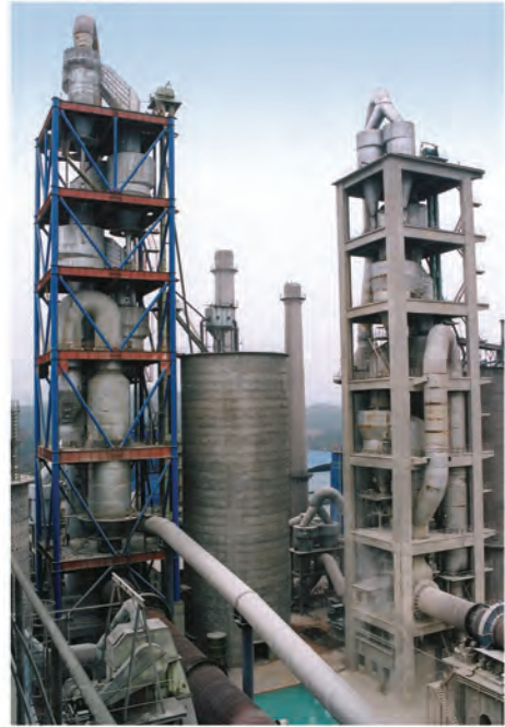
江山虎球水泥有限公司2000t/d熟料生产线 Jiangshan Huqiu Cement Corporation 2000t/d clinker production line
