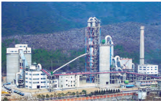
皖维高新材料股份有限公司 综合利用电石渣干磨干烧1000t/d熟料生产线 Dry grinding and dry burning 1000 t/d clinker production line with comprehensive use of calcium carbide dregs at Wanwei High & New Materials Co.,Ltd.
