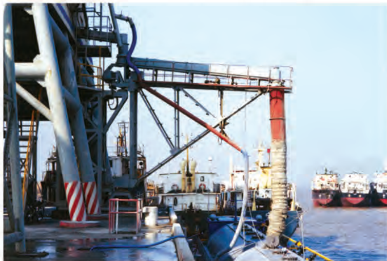
江苏京阳水泥有限公司水泥散装码头装船系统 Ship Loading System for Bulk Cement on river dock at Jiangsu Jingyang Cement Co.,Ltd
