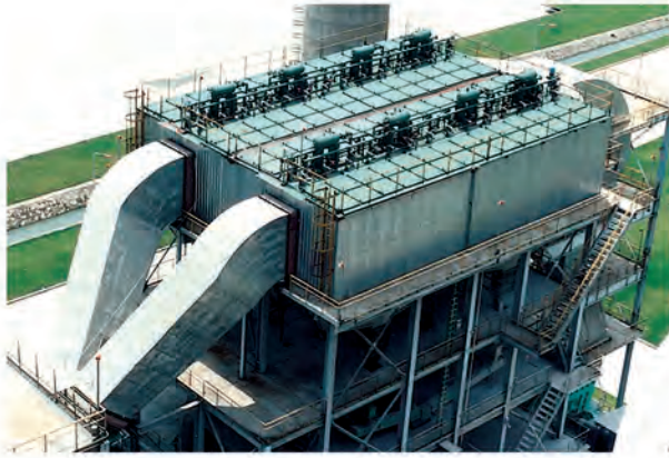
用于芜湖朱家桥70万吨粉磨系统 45万m 3 /h风量的气箱脉冲袋收尘器 A plenum pulse dust collector, air volume 450,000 m 3 /h at Wuhu Zhujiqiao Grinding Plant
