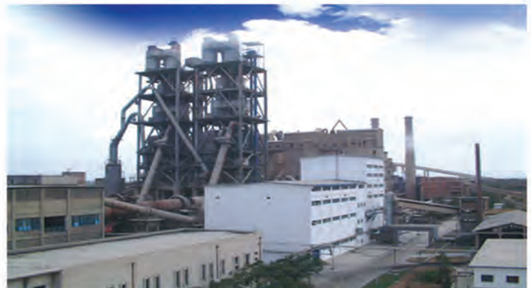
鲁南水泥厂两条2500t/d熟料生产线技改工程 Lunan Cement Plant 2500t/d clinker technical conversion production line
