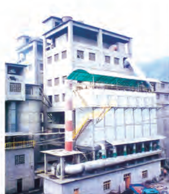
用于南京青龙山水泥厂烘干机收尘LFEF358-7 LFEF358-7 Bag Dust Filter Used at Qinglongshan Cement Plant
