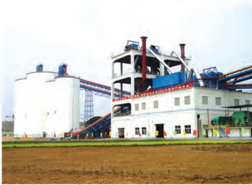
山东青岛年产150万吨水泥粉磨站 1,500,000 tons cement grinding plant at Qingdao Shandong
