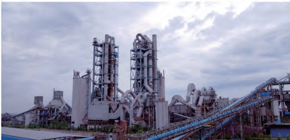
南阳航天水泥厂6000t/d熟料生产线及3000t/d熟料生产线 6000t/d and 3000t/d Clinker Production lines at Nayang Cement Corporation
