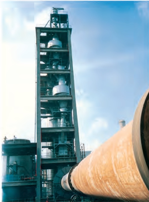
大田水泥厂600t/d熟料 国内首条国产化无烟煤煅烧生产线 600 t/d clinker production line at Datian Cement Plant, the first production line using anthracite as fuel in China
