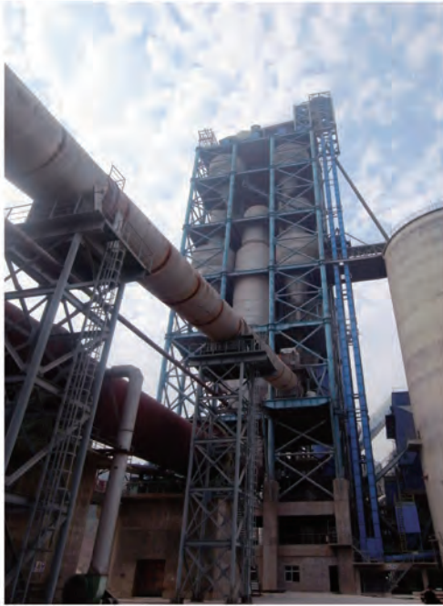
陕西众喜水泥公司5000t/d熟料生产线 Shanxi Zhongxi Cement Corporation 5000t/d clinker production line
