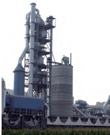
河北天福水泥有限公司3000t/d熟料生产线 3000 t/d Clinker Production Line at Tianfu Cement Company in Hebei
