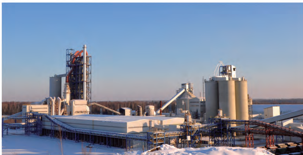
俄罗斯LSR集团水泥公司5000t/d熟料生产线 5000t/d Clinker Production line at LSR Corporation Cement Company Russia
