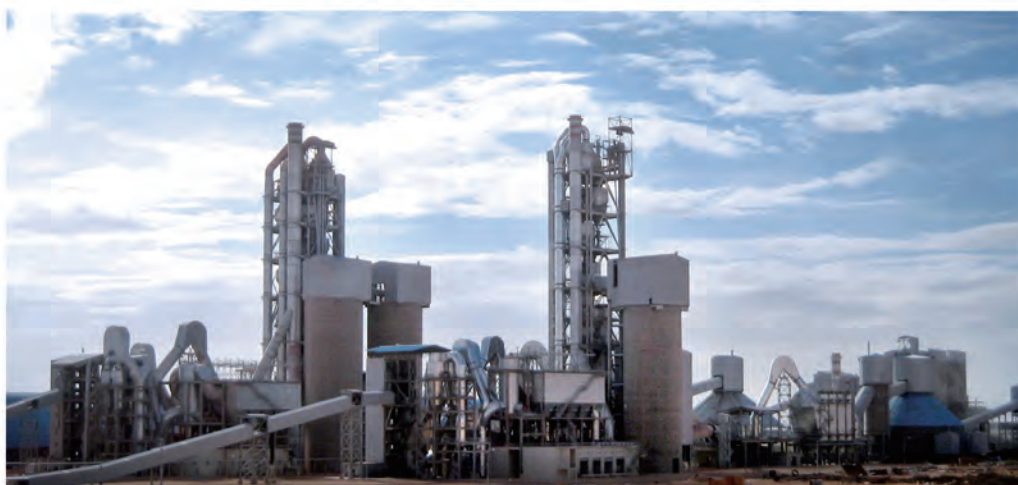
沙特阿拉伯Najran水泥有限公司6000t/d及3000t/d熟料生产线 6000t/d and 3000t/d Clinker Production lines at Najran Cement Company Ltd. Saudi Arabia
