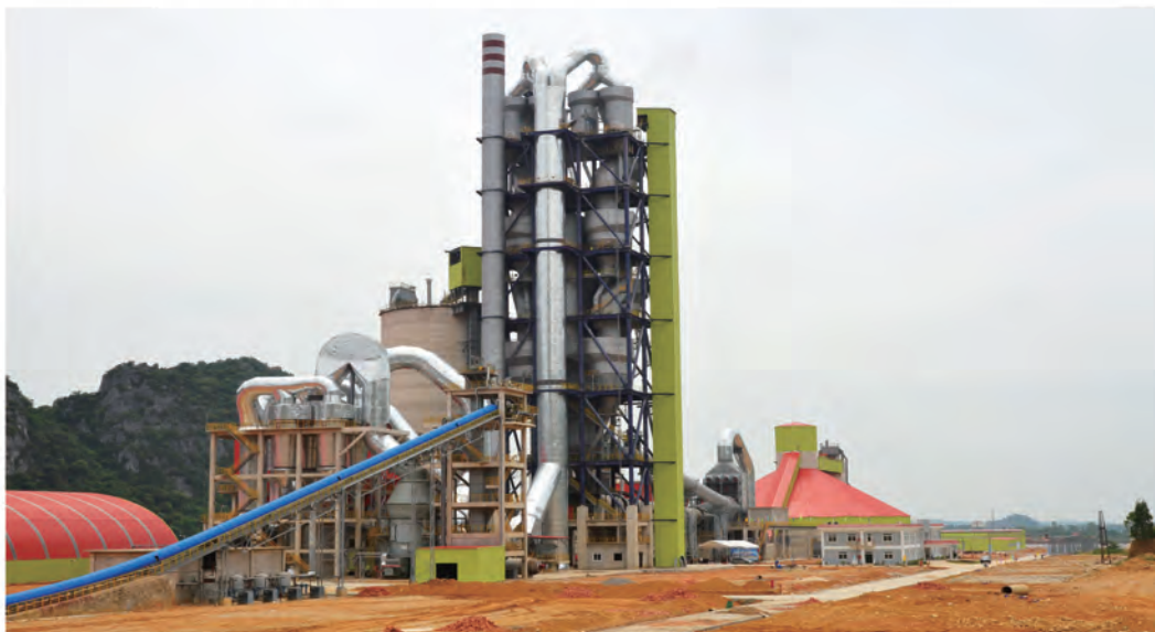
越南广福水泥有限公司5000t/d熟料生产线 5000t/d Clinker Production Line at Quang Phuc Cement Company Limited Vietnam
