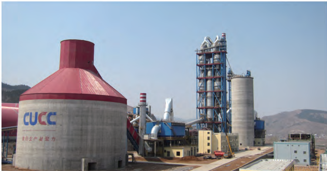
山东新泰中联泰丰水泥有限公司4000t/d熟料生产线 4000t/d Clinker Production Line at CUCC Taifeng Cement Company Limited in Xintai, Shandong
