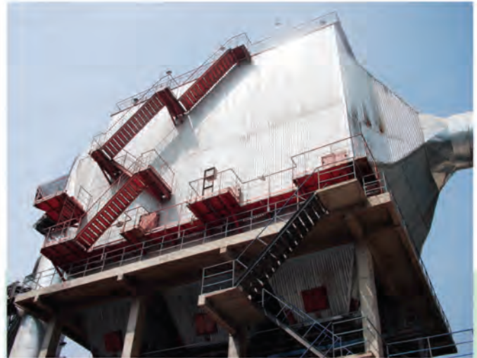
用于内蒙古冀东水泥有限责任公司5000t/d生产线窑头电收尘CDPK-E, 240m 2 240m 2 , Model CDPK-E Electrostatic Precipitator Used at Jidong Cement Co., Ltd Inner Mongolia
