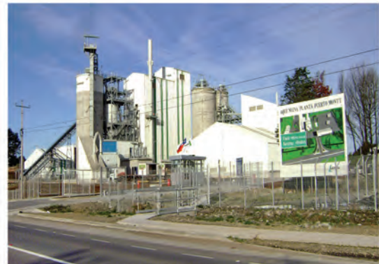
拉法基智利Puerto Montt水泥粉磨站 Lafarge Chile Puerto Montt Cement Grinding Plant
